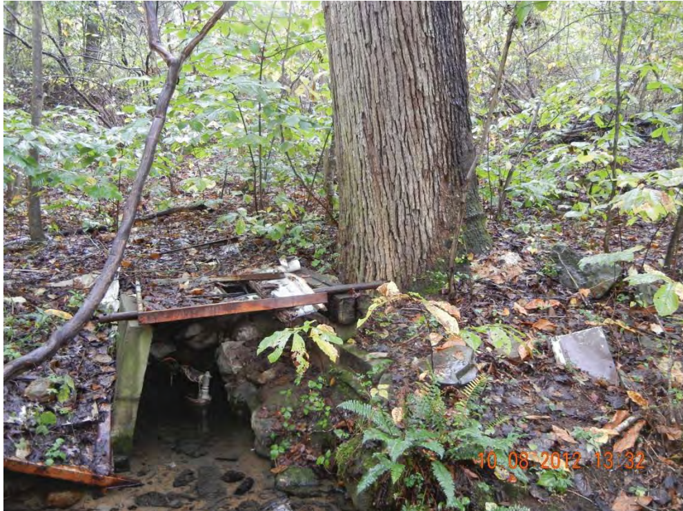
Photograph 13 – DSCN6993. N36.4923°, W-82.4624°. View of SPG-3 / STR-5 origin facing upstream and east near STA 2842+50R.
