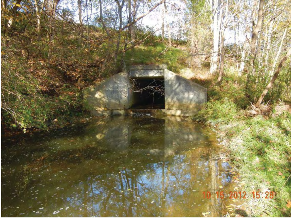
Photograph 21 – DSCN7211. N36.5060°, W-82.4341°. View of STR-8 facing upstream and north at outlet of existing structure beneath I-81 at STA 2940+20R.
