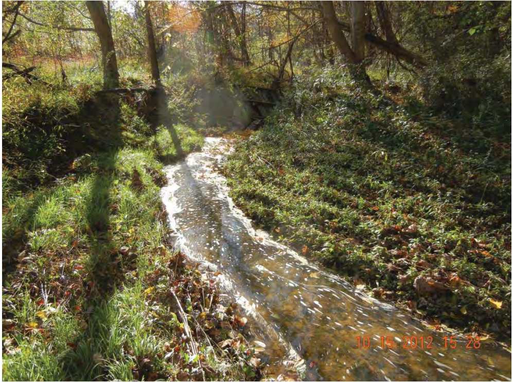
Photograph 22 – DSCN7212. N36.5060°, W-82.4341°. View of STR-8 facing downstream and south at outlet of existing structure beneath I-81 at STA 2940+20R.
