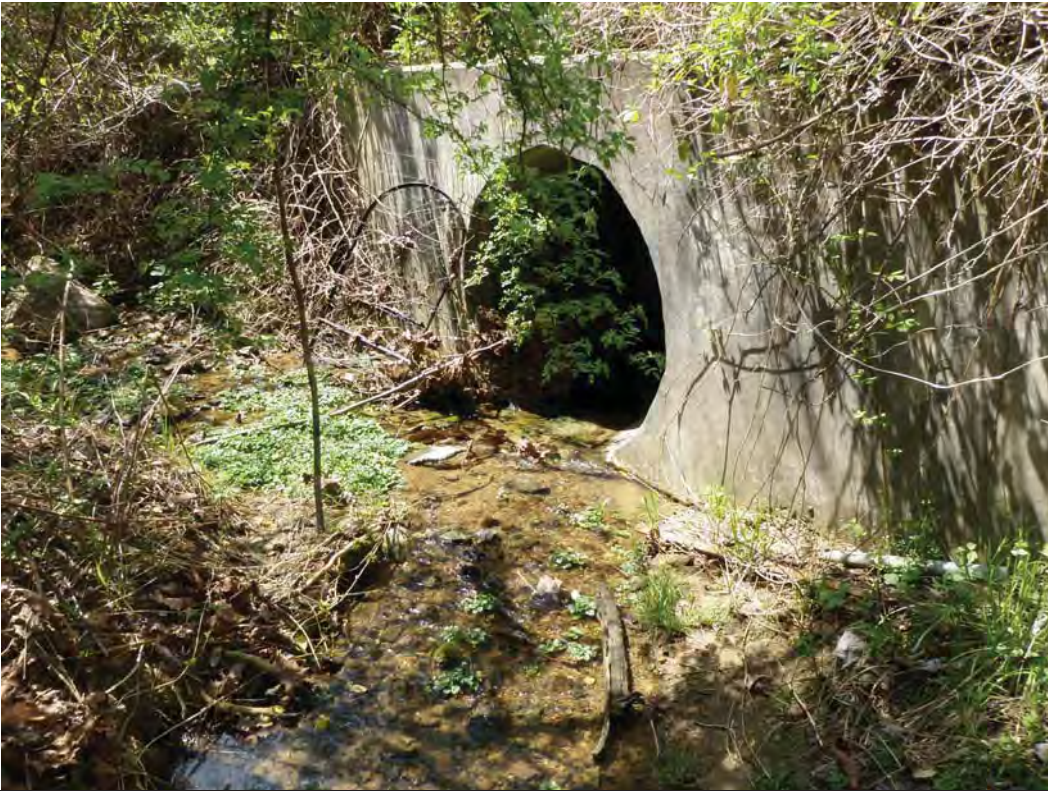
Photo 9: Downstream view of STR-9 at inlet of pipe under Rocky Branch Road. SPG-4 flows in from left in photo.
