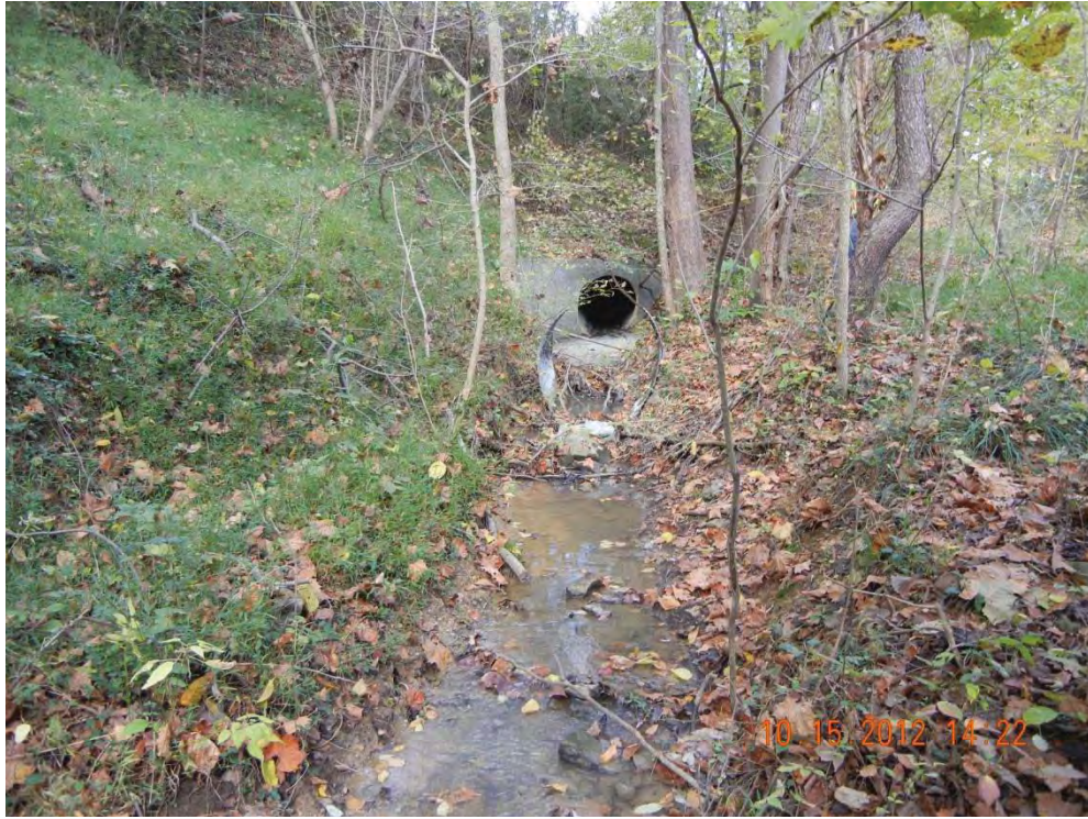
Photograph 17 – DSCN7189. N36.5030°, W-82.4439°. View of STR-7 facing upstream and northeast at culvert outlet beneath I-81 at STA 2909+50R.
