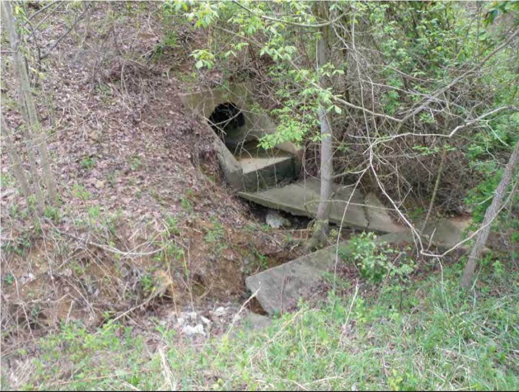
Photo 1: WWC-1 at outlet of pipe at Sta. 2868+50.
