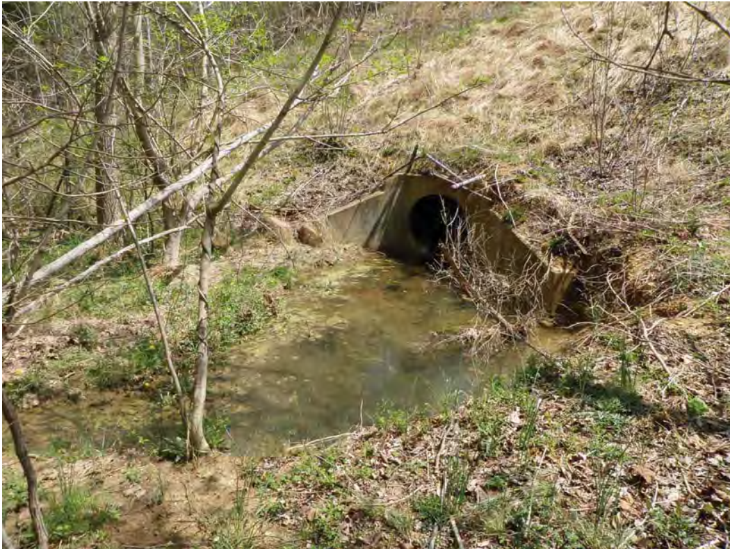
Photo 4: Outlet of pipe at Sta. 2881+25 that carries WWC-2.
